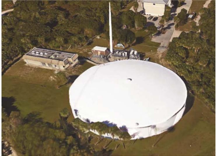
As is common with many water utilities, Punta Gorda was having difficulty maintaining optimal chlorine residuals for water disinfection in their distribution system. After pursuing common operational strategies such as tank flushing, operating at lower tank levels to reduce water age and distribution line flushing, the utility staff decided to employ a Tank Shark® mixing system in the larger 2 MG Punta Gorda Isles tank.
