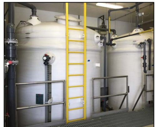
400 Pound Per Day Microclor™ system skid (left) and Hypo Storage tanks (right). Also includes 40 ton Salt Brine tank not shown.
