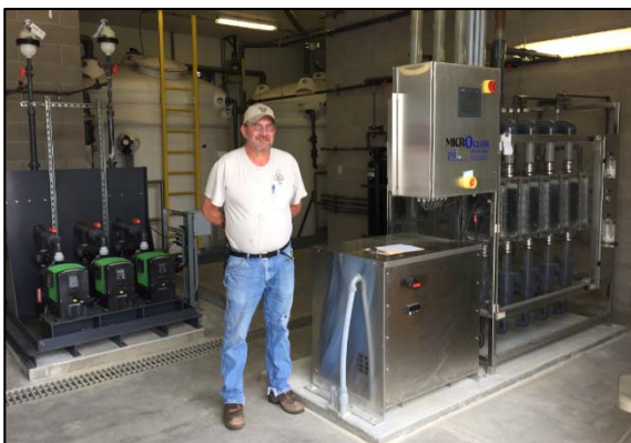
400 Pound Per Day Microclor™ system skid (left) and Hypo Storage tanks (right). Also includes 40 ton Salt Brine tank not shown.
