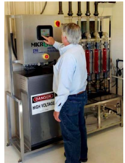
Daphne Utility operators adding salt and operating the Microclor™ OSHG
