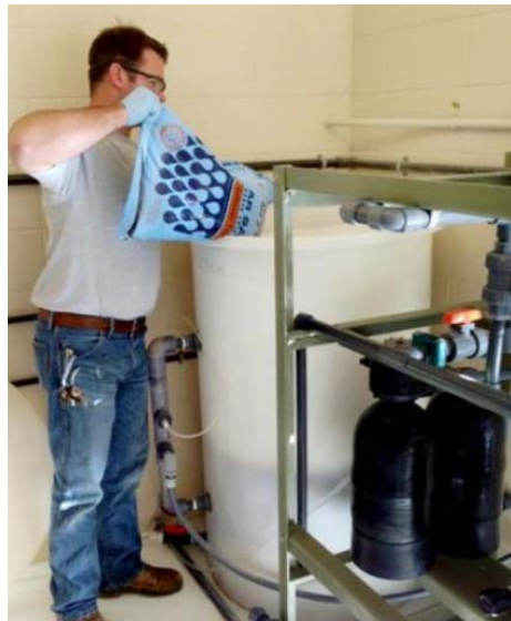
Daphne Utility operators adding salt and operating the Microclor™ OSHG
