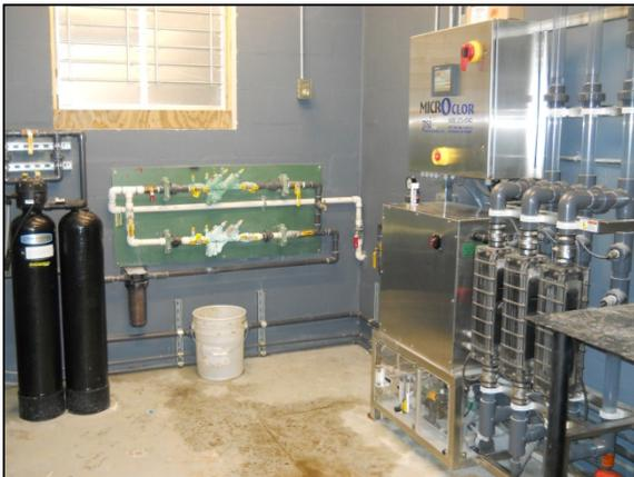
**Process Solutions, Inc.'s MicrOclor™ MC-60 On-Site Hypochlorite Generation System**
