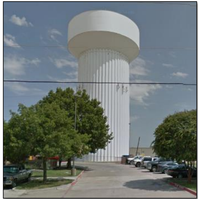
1.5 MG Southwestern Tank – Tower 1
