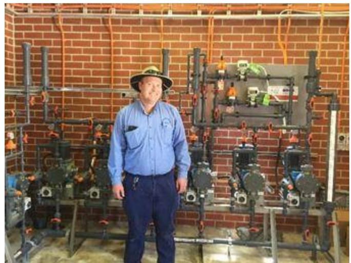
*Encore® 700 diaphragm chemical dosing pumps*
