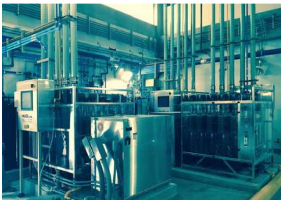
Three 1,500 PPD Microclor® OSHG skids
