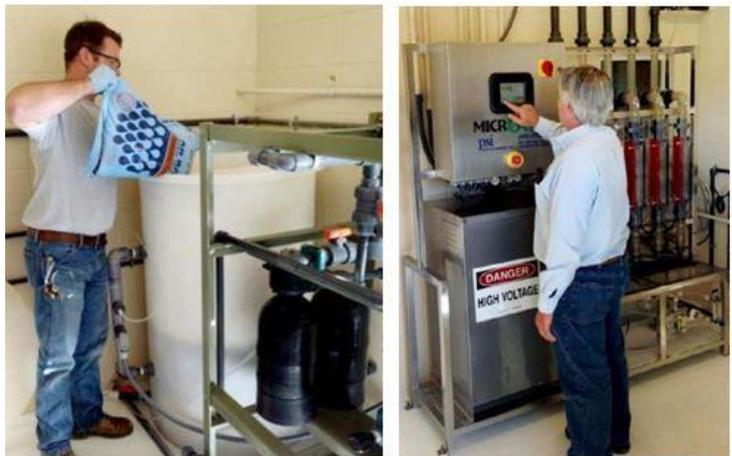
*Daphne Utility operators adding salt and operating the Microclor® OSHG*
