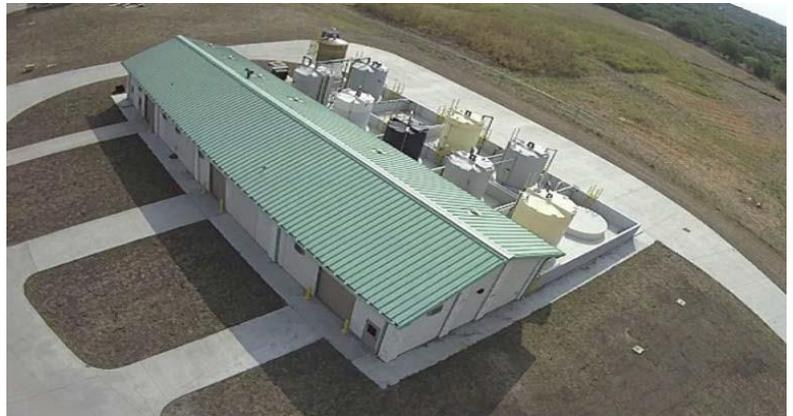
After observing the reliable vertical Microclor® system in Pine Bluff, Midlothian moved ahead to include a 1,200 lbs./day system in the design of the new plant. Installation was successful, with the general contractor preparing the piping and electric and setting and plumbing the unit. PSI’s technicians tested and commissioned the system and the new plant went live in July 2013.
