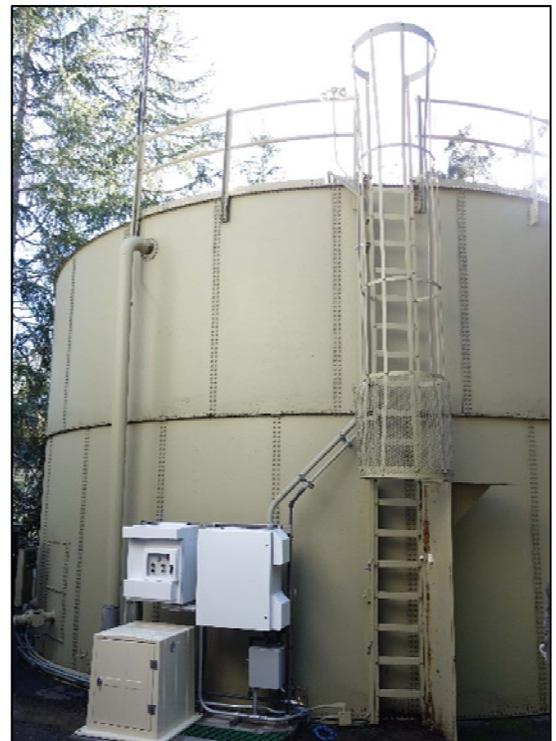
UGSI ChemLocker™ and Tank Shark® tank mixing and boosting system
